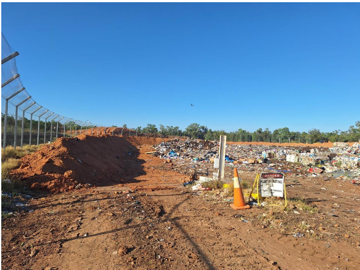
Figure 1: Current cell, recent earthworks
