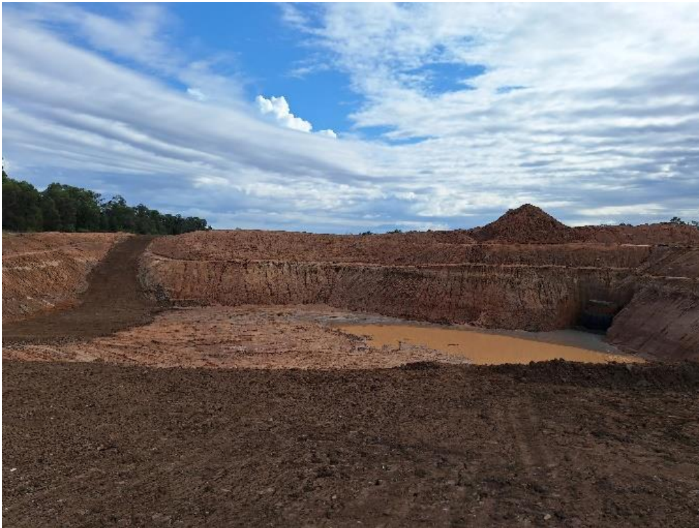
Figure 2: New cell works, including sump & machine access road
