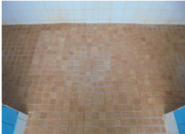
Figure 4. Remove existing tile bed
