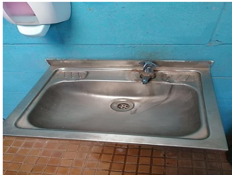
Figure 9. Remove existing wall basin
