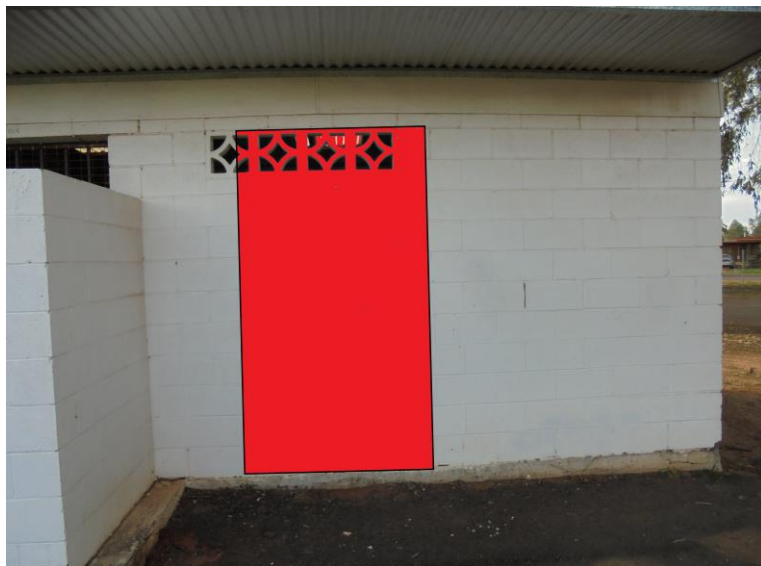
Figure 5. Doorway to be cut into Southern wall
