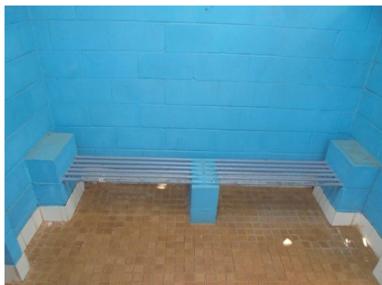
Figure 7. Demolish and remove existing bench seat
