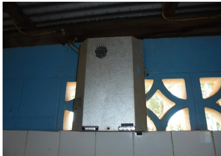
Figure 1. Remove existing instantaneous electric hot water systems
