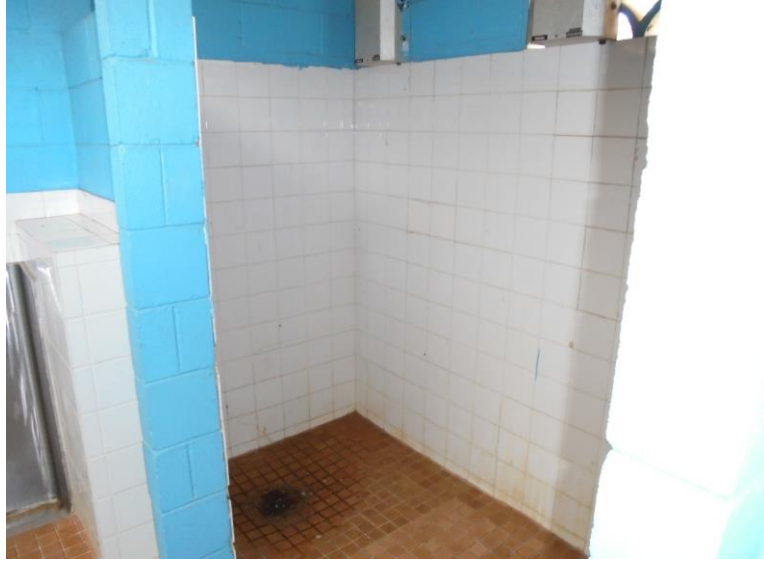
Figure 3. Remove existing wall tiles to shower
