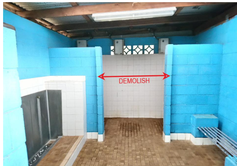
Figure 2. Demolition of two (2) Nib Walls
