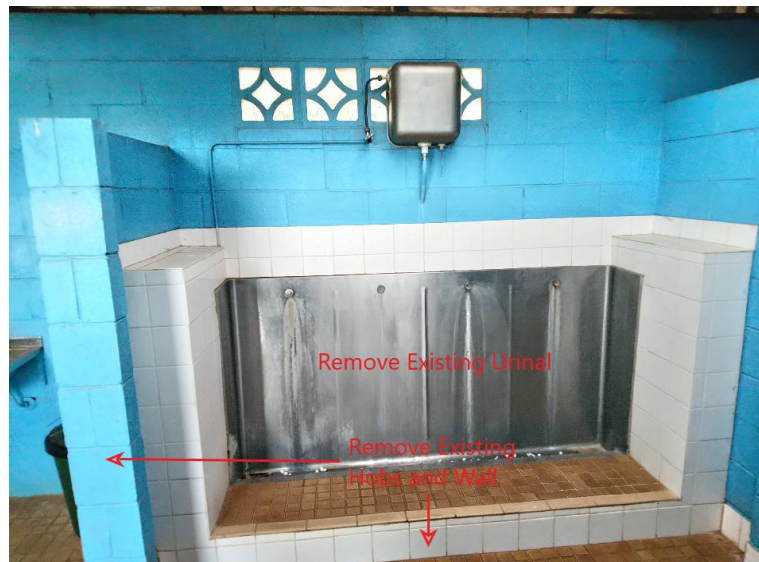
Figure 6. Demolish and remove existing Urinal, hobs and wall
