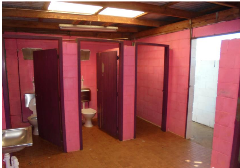
Figure 15. Demolish all existing cubicles
