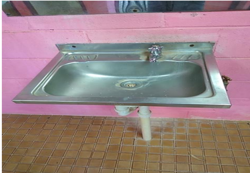
Figure 14. Remove existing wall basin
