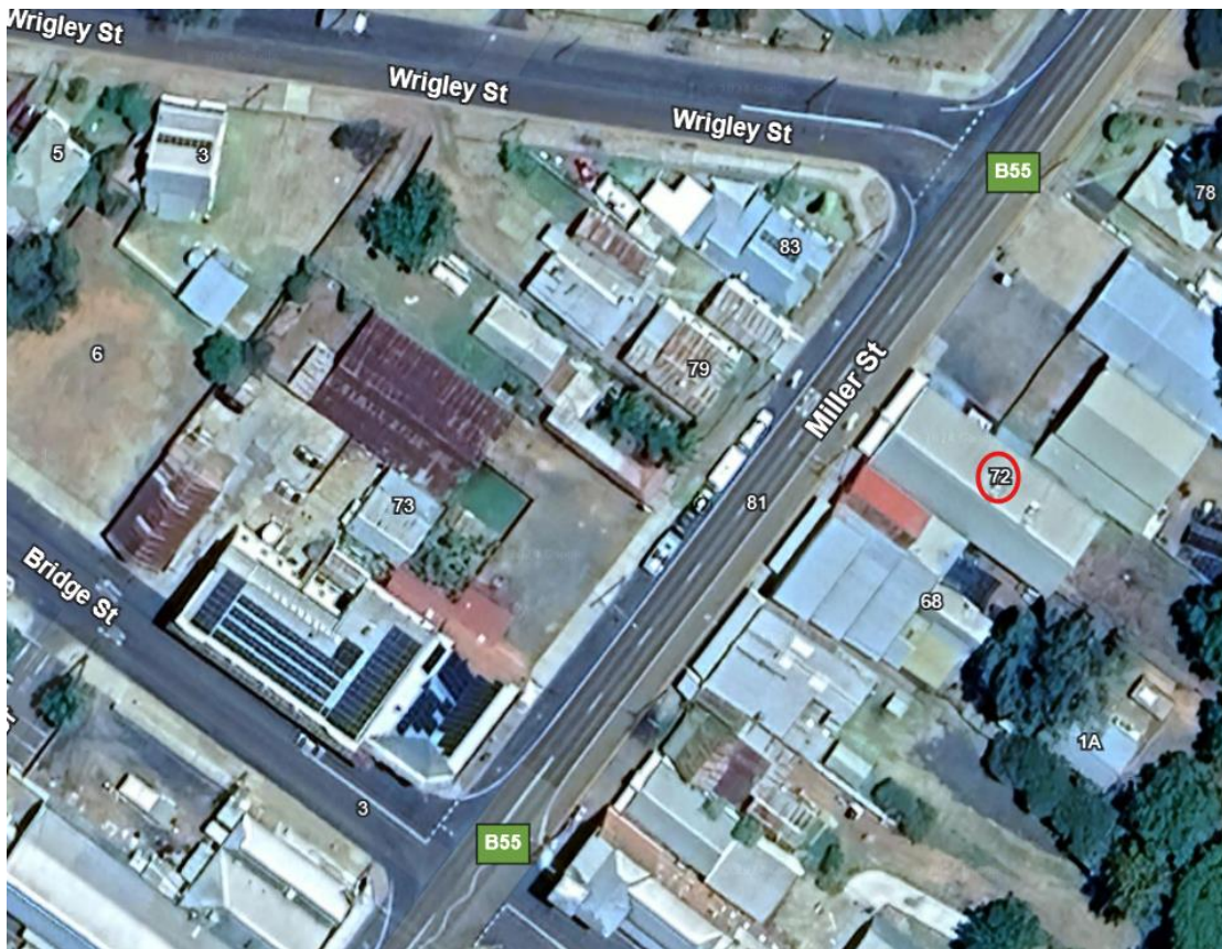
Figure 3: Aerial image of the site location
