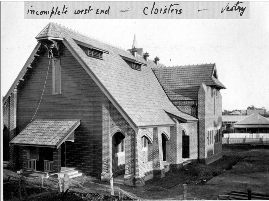
Figure 8: Northern Entry/ Narthex as originally built. The church was never extended beyond the chamferboard clad, temporary timber framed wall to this end of the church. (Source: St Ambrose archives)
