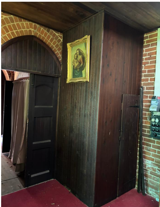
Figure 31: Spiral stair in Vestry to Loft above, enclosed within timber v.j. boards.
