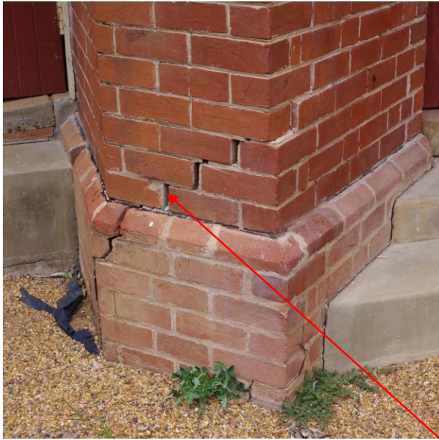
Figures 18 & 19: Substantial cracking to western and southern walls of church. (Source: Michael Scott)
