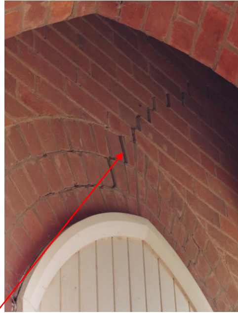
Figures 18 & 19: Substantial cracking to western and southern walls of church. (Source: Michael Scott)
