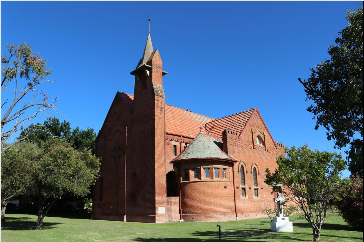
St Ambrose Memorial Church from the southeast.
