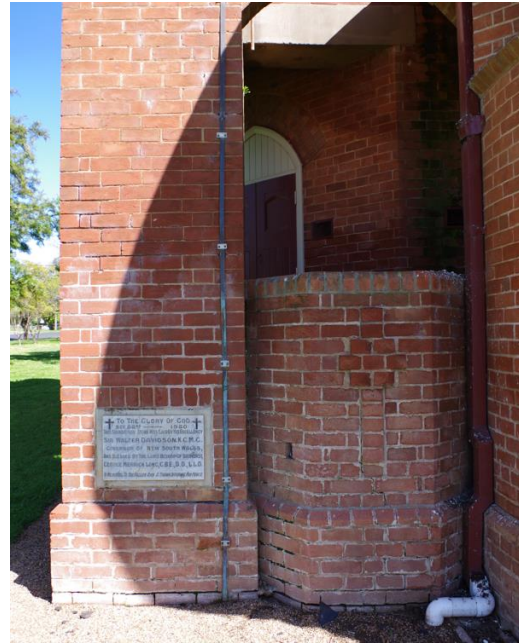
Figure 30: External brick pulpit to be removed and concrete floor behind.
