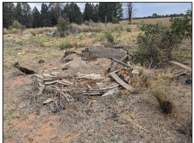
Water tank ruins
