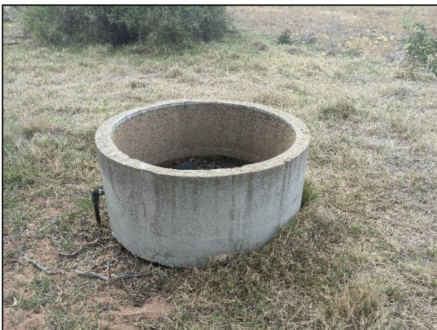
Water tank ruins
