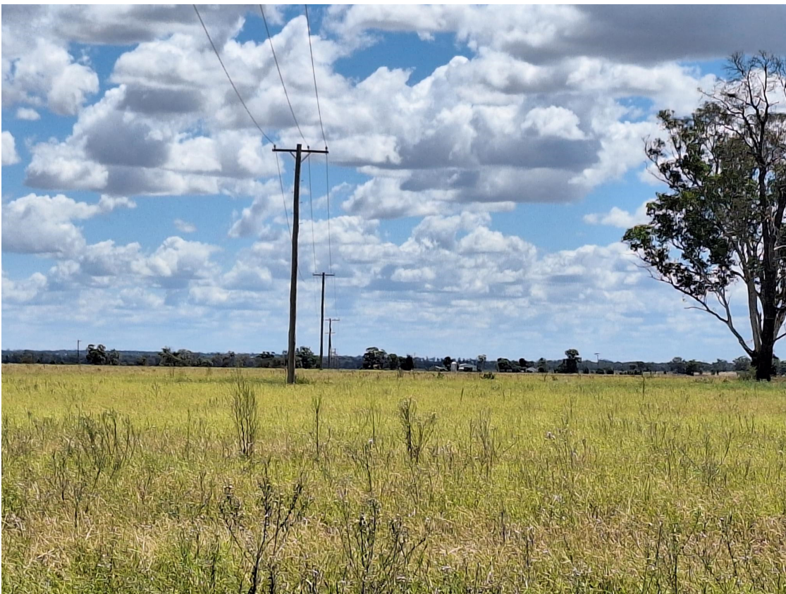
Plate 7: An 11 kV power line located in a 20-metre-wide easement crosses the subject land east to west
