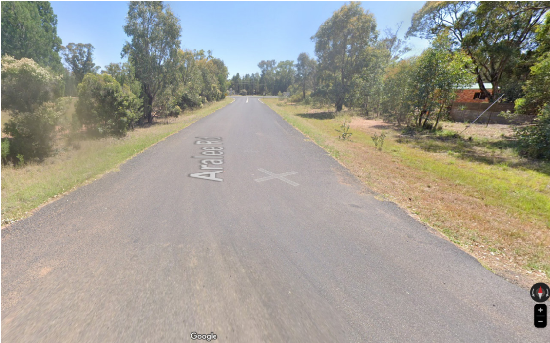
Plate 2: Aralee Road (sealed part) looking north to the Oxley Highway (subject land on left, residential development on right)
