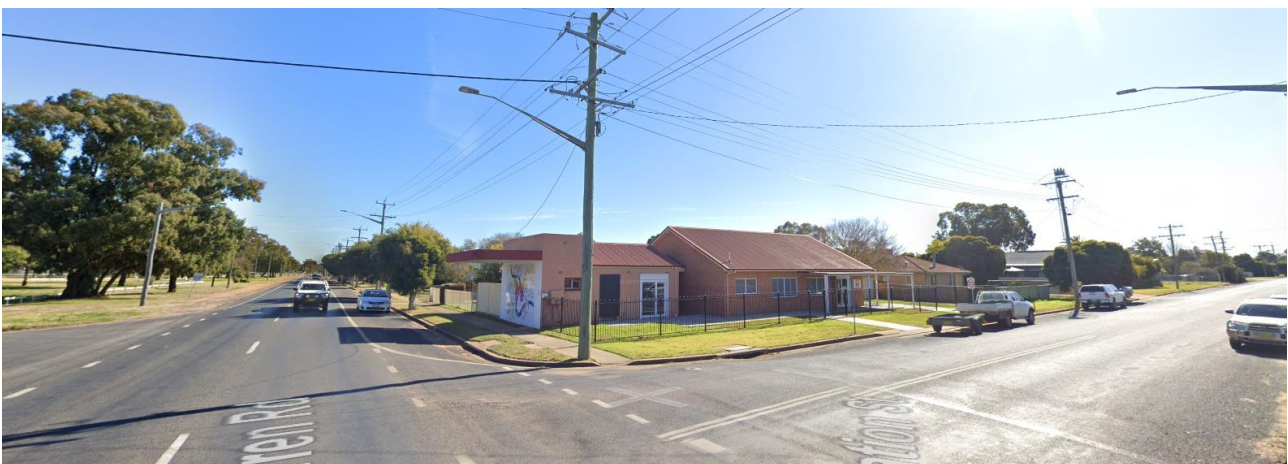
FIGURE 23. EXISTING CLIENT MEDICAL CLINIC AT 140 WARREN ROAD
