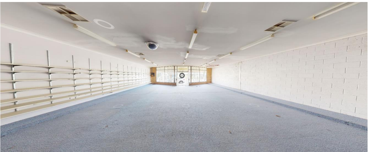
FIGURE 11. INTERIOR OF EXISTING BUILDING ON SUBJECT SITE, VIEW TO NORTH-WEST TOWARD MILLER ST
