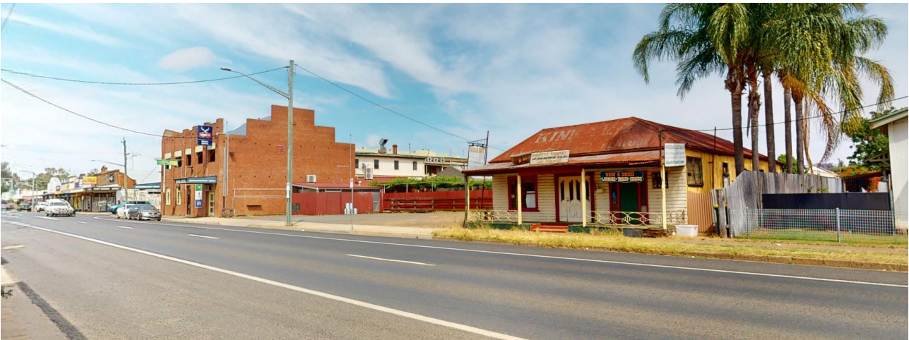
FIGURE 4. SINGLE STOREY BUILDING AT 77 MILLER STREET, DIRECTLY TO SOUTH-WEST OF SUBJECT SITE, VIEWED FROM MILLER ST
