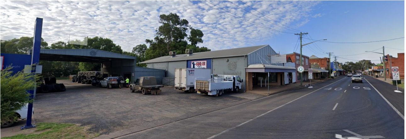
FIGURE 9. NORTH-WEST BLOCKWORK FAÇADE ALONG BOUNDARY WITH TYRE SHOP. EXISTING TYRE SHOP SIGNAGE CAN BE SEEN APPENDED TO FAÇADE
