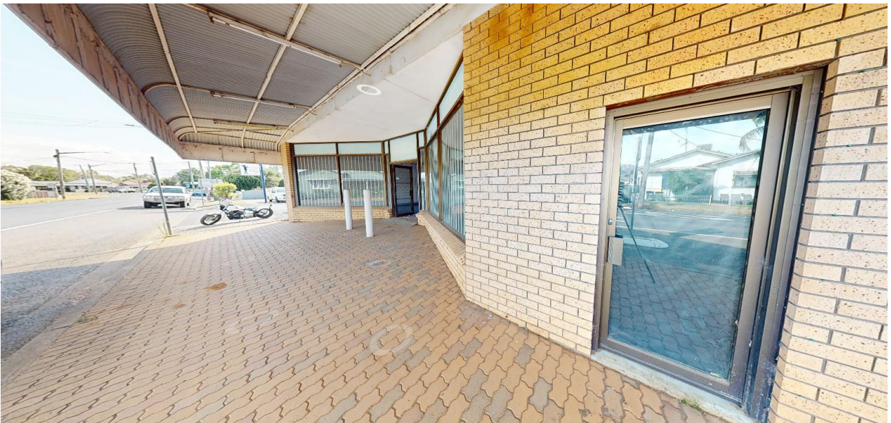
FIGURE 10. EXISTING SHOPFRONT ON SUBJECT SITE, VIEW TO NORTH FROM MILLER STREET
