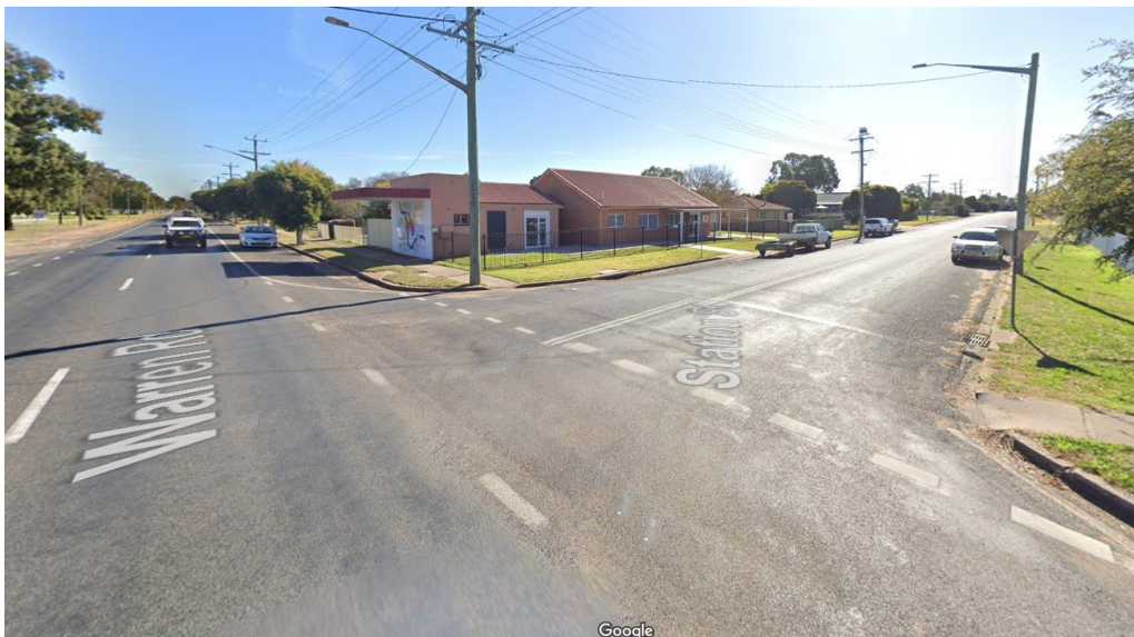
Figure 1 Existing Medical Centre at 140 Warren Street Source: Google Maps (2022)
