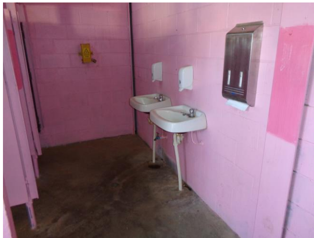
Figure 27 Remove Existing Wall Basins
