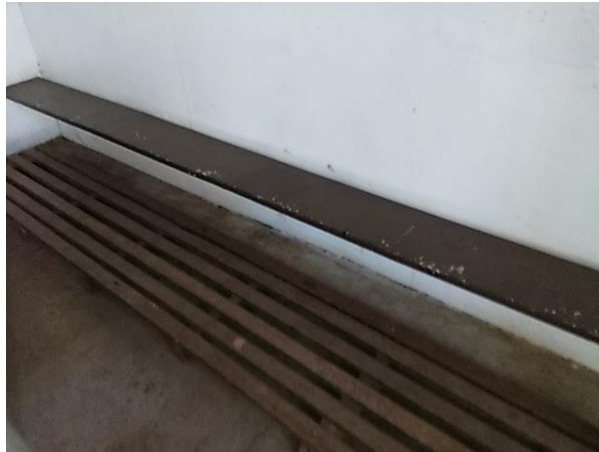
Figure 1 Remove and replace bench seating
