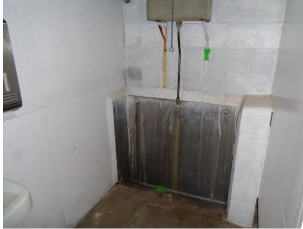
Figure 3 Remove and Replace Existing Urinal
