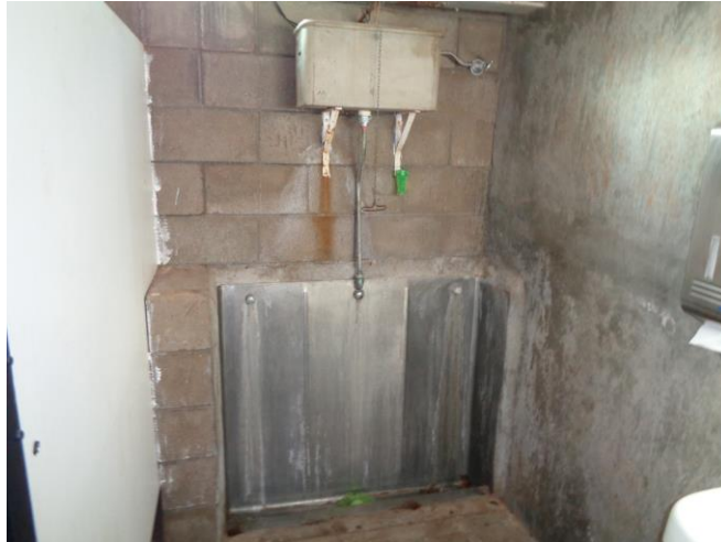
Figure 11 Remove and Replace Existing Urinal
