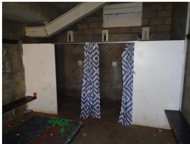
Figure 14 Remove compressed cement sheet return walls
