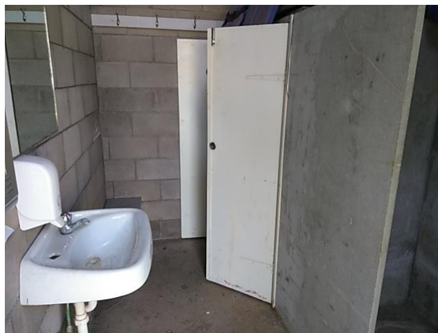
Figure 22 Remove and Replace Existing Wall Basin Tapware
