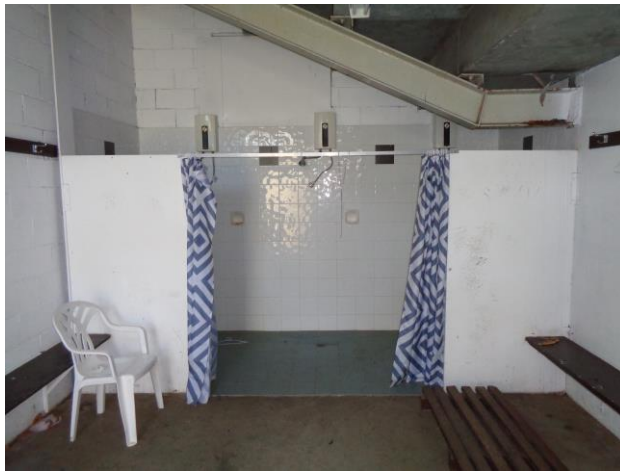
Figure 6 Remove compressed cement sheet return walls
