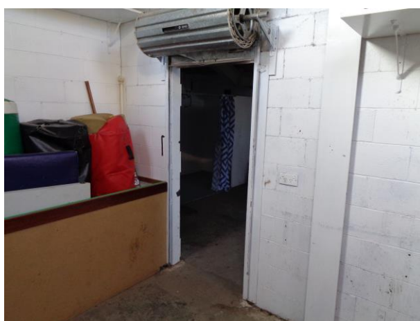
Figure 17 Remove shutter and install hinged door
