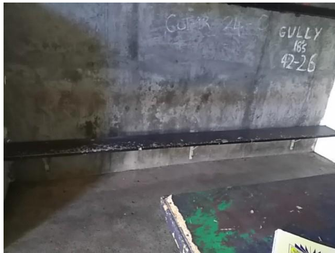
Figure 9 Remove and replace bench seating
