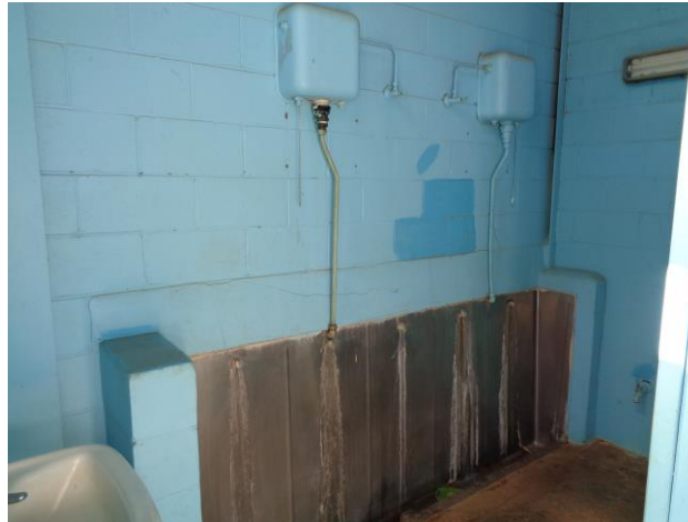
Figure 25 Remove Existing Urinal and Cisterns
