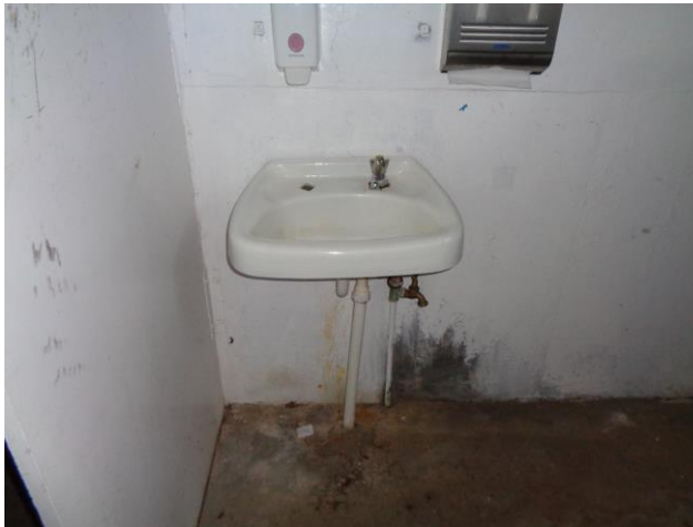
Figure 4 Remove and Replace Existing Wall Basin and Tapware
