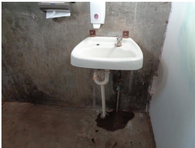
Figure 12 Remove and Replace Existing Wall Basin and Tapware
