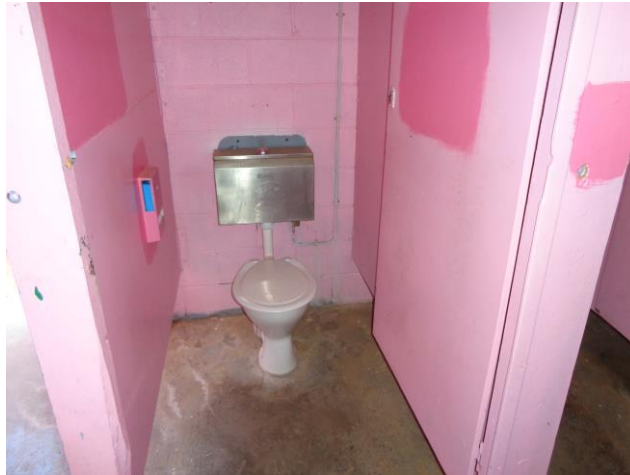
Figure 26 Remove Existing Toilet Suites and Toilet Cubicles
